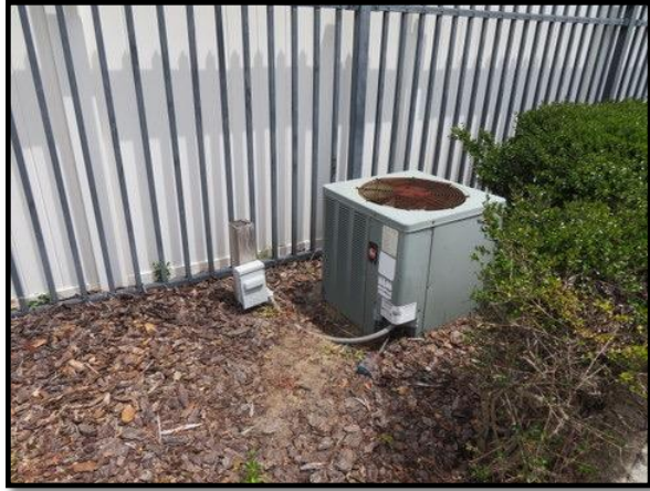
Figure 1 – Split System Condensing Unit
