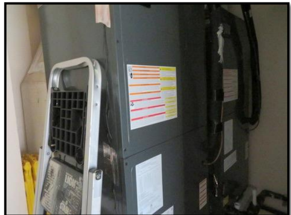
Figure 2 - Split System Air Handling Units
