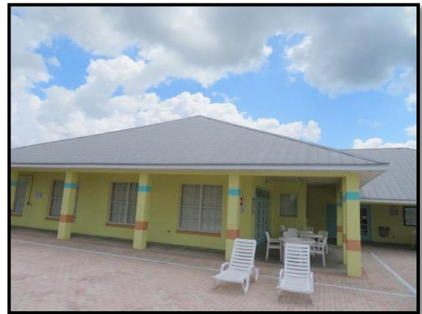
Figure 2 – Clubhouse Rear Elevation
