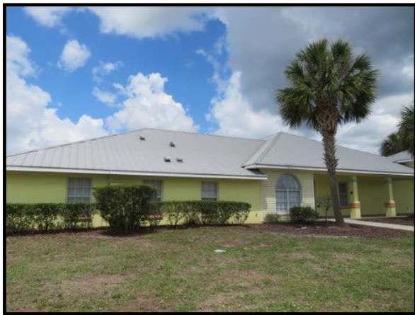
Figure 1 – Clubhouse Rear Elevation
