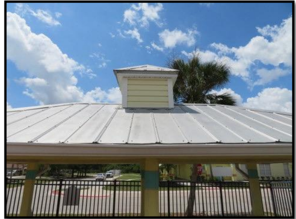
Figure 2 – Playground Pavilion Roof
