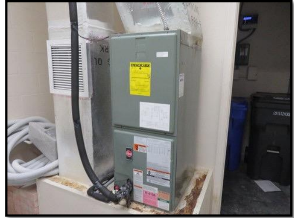
Figure 2 - Split System Air Handling Unit
